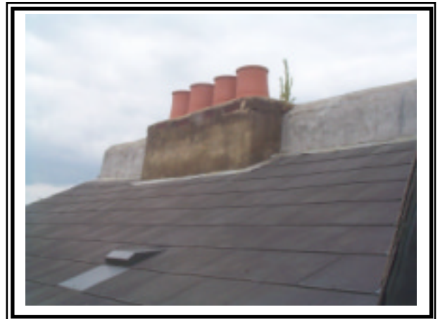
Photo 8 – Back addition roof/chimney stack
